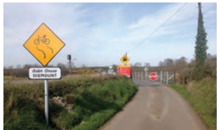
Typical Rural Level Crossing.
